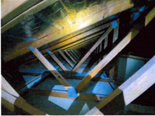
Showing inside roof void.
