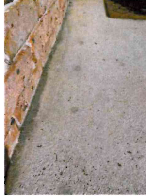
Shows drill holes indicating a previous treatment however no details available.
