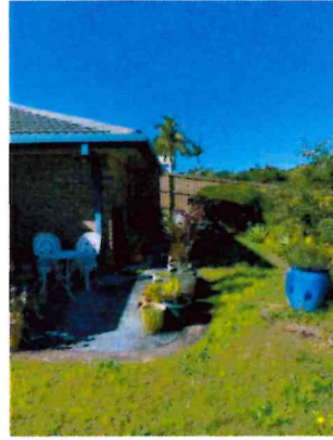
Showing rear of dwelling.
