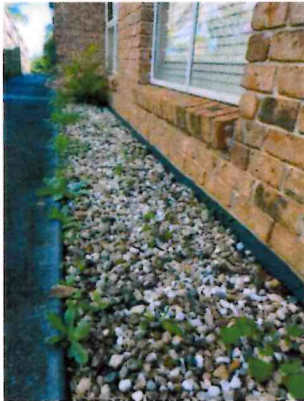
Showing exposed slab edge.
