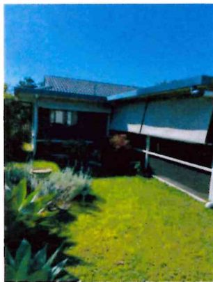
Showing rear of dwelling.
