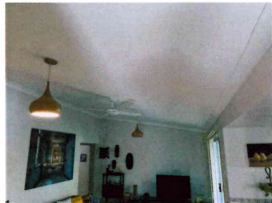
Showing internal roof structure.
